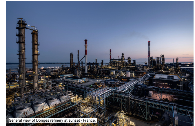
General view of Donges refinery at sunset - France.
